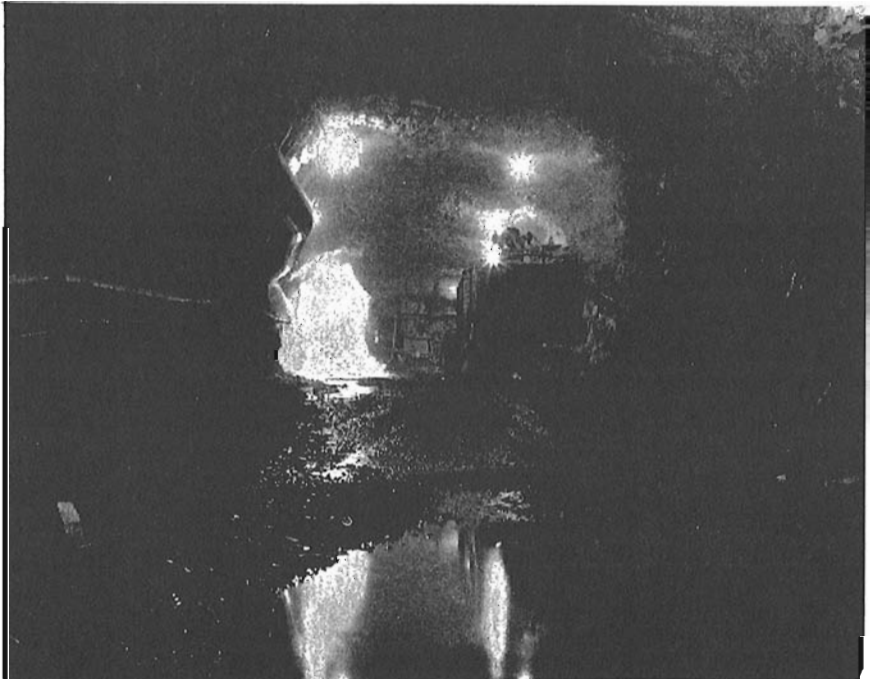
FIRST CONTRACT — tunnel between Jarry and Jean-Talon Streets under Berri Street.
