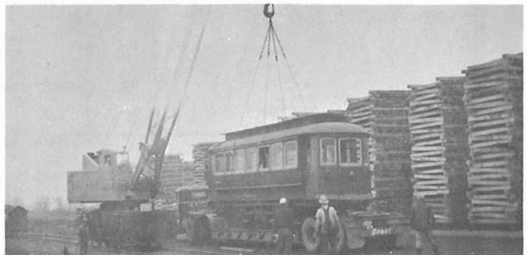
The above two photographs by Fred Angus, show the arrival at Delson of No.6 from Ottawa, and its transfer from highway trailer to rails close to the Museum Site.
