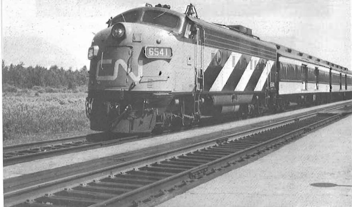
Canadian National 6541 on Train 27 at Morrisburg Ont. on 16 August, 1965. CN's practice of mounting the bell on the cab roof of passenger and freight A-units is ably demonstrated in this photograph. The normal position of the bell on such locomotives is near the front truck under the pilot where it unfortunately is susceptible to being clogged with snow.
