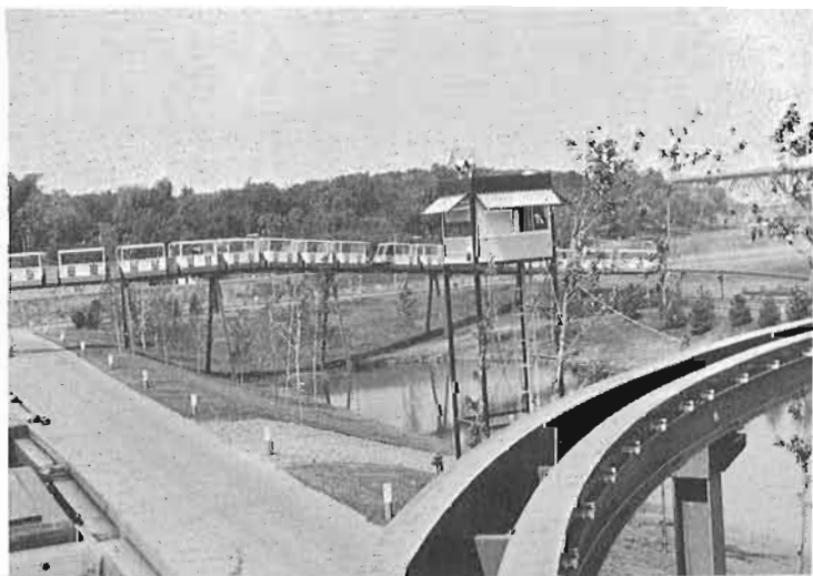
The switch and shop lead as seen from a passing train.
