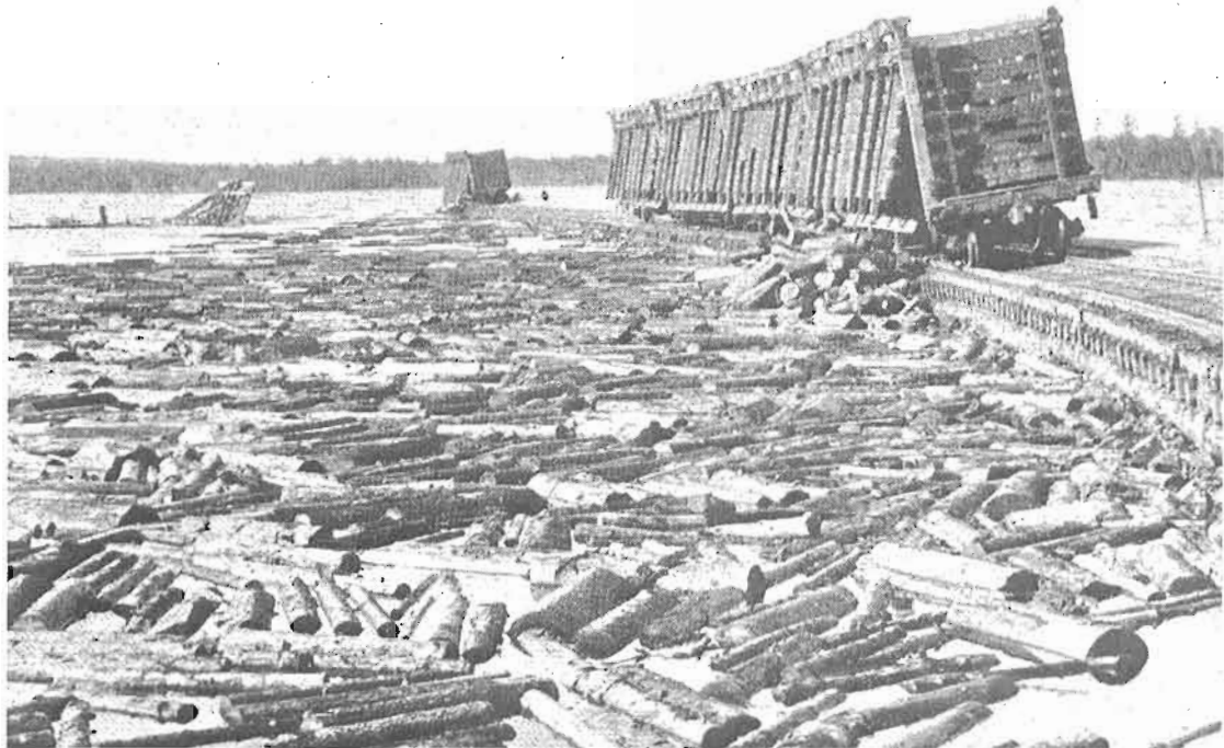
photo above Southern terminus of Eagle Lake and West Branch Railroad at Umbazooksus Lake. Hinged-sided cars dump 12\frac{1}{2} cords of wood into the lake from the 600 foot long sloped trestle. Photo courtesy of L.B. Walker, Salem, Mass.
