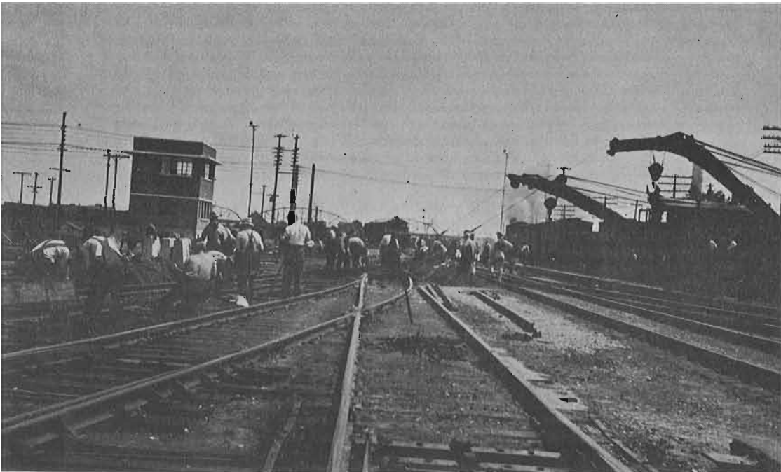
RUGBY JUNCTION on the C.P.R. was rearranged in July of 1947. The track gang was replacing the crossovers, after the new tower on the north side was built. The over-bridge in the distance is the Arlington Street bridge which spans the yards at that point.
