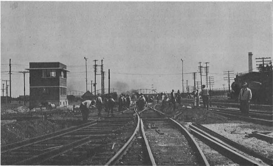
RUGBY JUNCTION on the C.P.R. was rearranged in July of 1947. The track gang was replacing the crossovers, after the new tower on the north side was built. The over-bridge in the distance is the Arlington Street bridge which spans the yards at that point.
