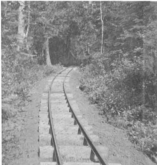
The well-located but temporarily unballasted main line of the Algoma Eastern Miniature Railroad winds through the woods near "West Lakehead".
