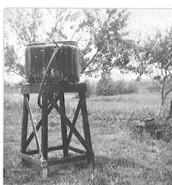
The water-tank, once a washing-machine body (?) on the Happy Valley Railway.
