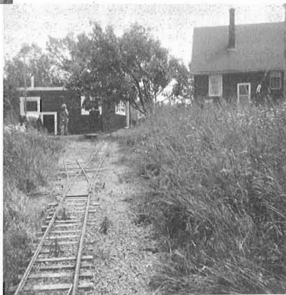
Looking east along the HVRR main line, towards the engine house. One of the neighbours is observing the lighting-up operation. The main switch to the yard appears in the foreground.
