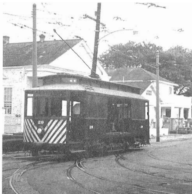
↑ RAIL-GRINDER CAR 29 OUTSIDE THE CARROLLTON Carhouse. Note filled inner tracks in the foreground, evidence of NOPSC's dual-gauge operation, over the years.
