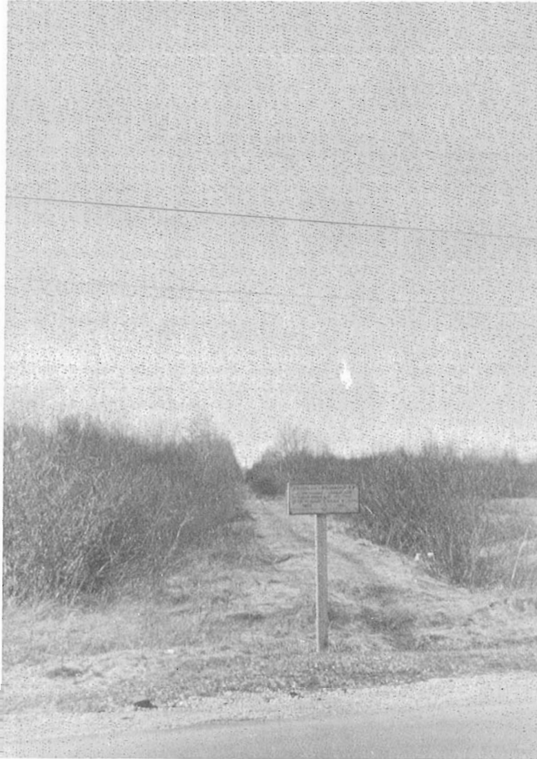
↑ RIGHT-OF-WAY OF THE CHAMPLAIN AND ST. LAWRENCE RAIL ROAD, AS IT AP- peared in 1967, looking east from Highway 9-A towards l'Acadie. The marker was erected by the Canadian Railroad Historical Association about 1936 and indicates that the derelict roadbed is that of Can- ada's first public railway. Photo courtesy S.S.Worthen.
