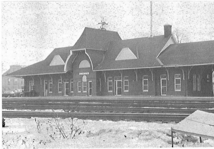
↑ CANADIAN NATIONAL RAILWAYS STATION AT ST-HYACINTHE, Québec, was built about 1899 by the Grand Trunk Railway Company of Canada. It is of brick construction and is in good condition. In design, it resembles other CN stations at Richmond and Sherbrooke, Québec. Ken Goslett took this photo on 4 February, 1973.
