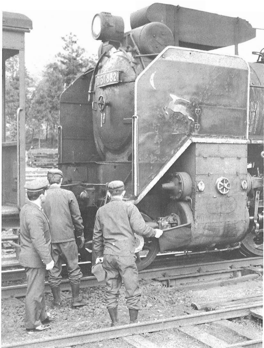
THE TRAIN CONDUCTOR- ON THE LEFT WEARING THE UNIFORM CAP - SUPERVISES the uncoupling of a D 51 helper in Tsuge yard on the JNR's Kansai line. The yardman on the right signals the engineman with a green flag to back off. D 51 882, paint pitted, bearings worn, leaking steam, carries a few cosmetic touches - an effort to hide all too obvious deterioration. Jumping deer on smoke deflectors and crimson main rods are non-standard, certainly the work of an artistic shop staff. In service as a helper between Kameyama and Tsuge, the D 51 is assigned to Nara, where deer roam the suburbs, which may explain the artistic touches.
