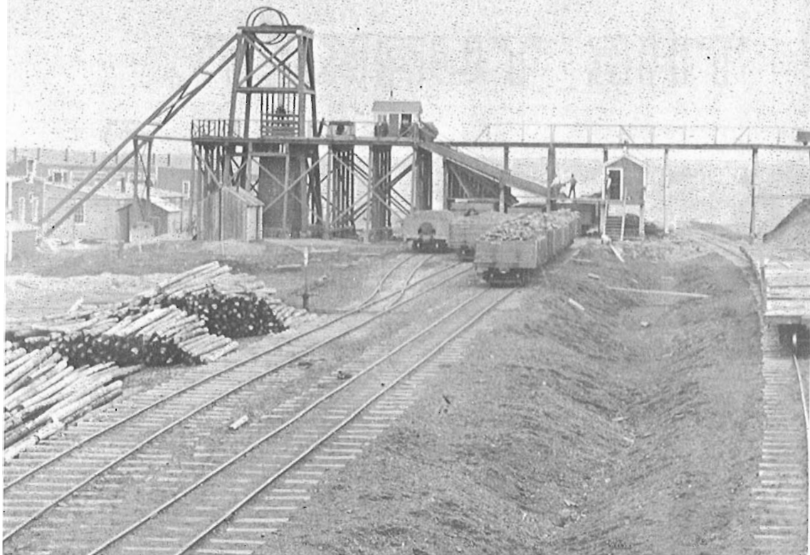
↑ THE HEAD-FRAME OF NUMBER 1 SHAFT OF THE GALT COAL MINES AT LETH- bridge, Alberta, about 1890. The roundhouse of the North West Coal & Navigation Company is in the right background.
