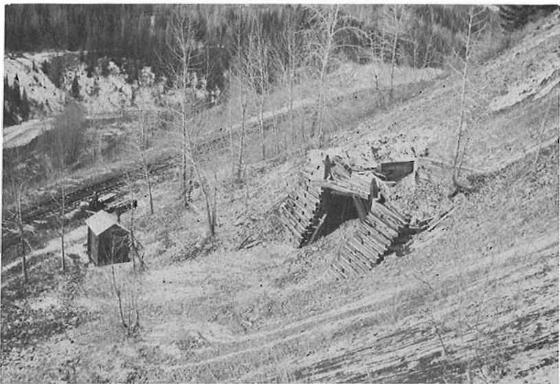
THE SOUTH PORTAL OF LOOP TUNNEL: THE LOWER LINE AT MILE 8 CAN BE SEEN among the trees immediately above the peak of the shed roof, on this side of the creek. Photo by the Author.
