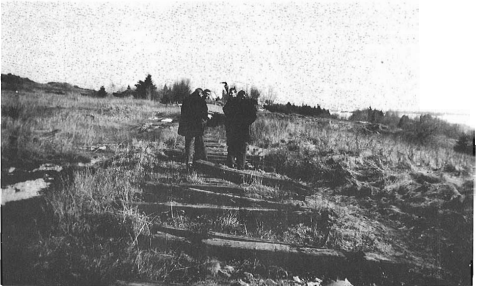
IN THE SPRING OF 1955, A GROUP OF RAILWAY-ARCHEOLOGISTS WERE WALKING along the abandoned roadbed, east of the original stamp-mill of the Bruce Copper Mines, towards the loading docks of the trap-rock company. Photo courtesy of the Author.
