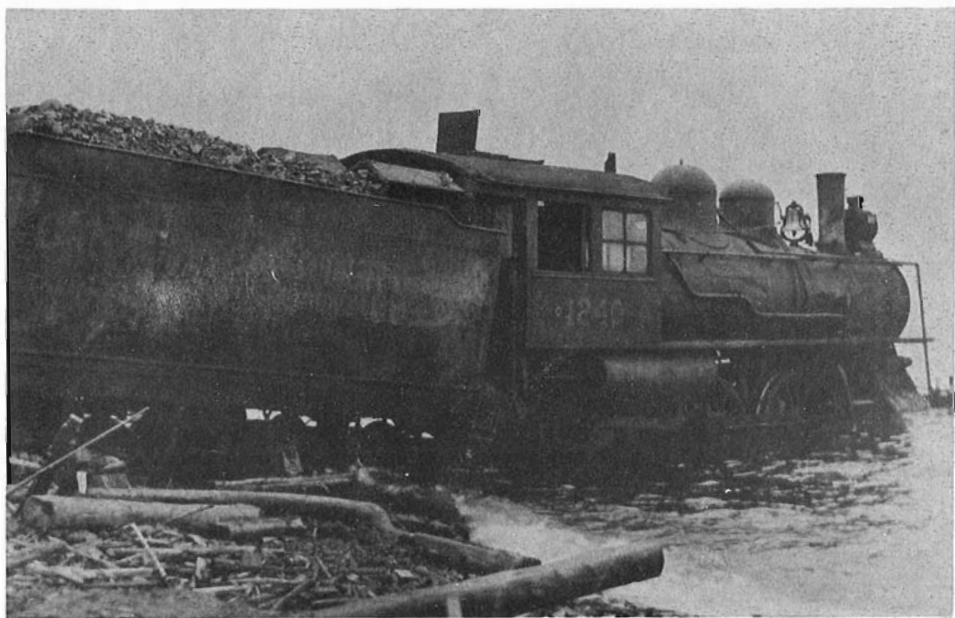
Construction scenes along the Canadian Northern Railway include this un-identified 4-6-0 with gantry on the Blende River Bridge following its completion. No. 1240 got her feet wet following a wreck at the Current River Yard,
