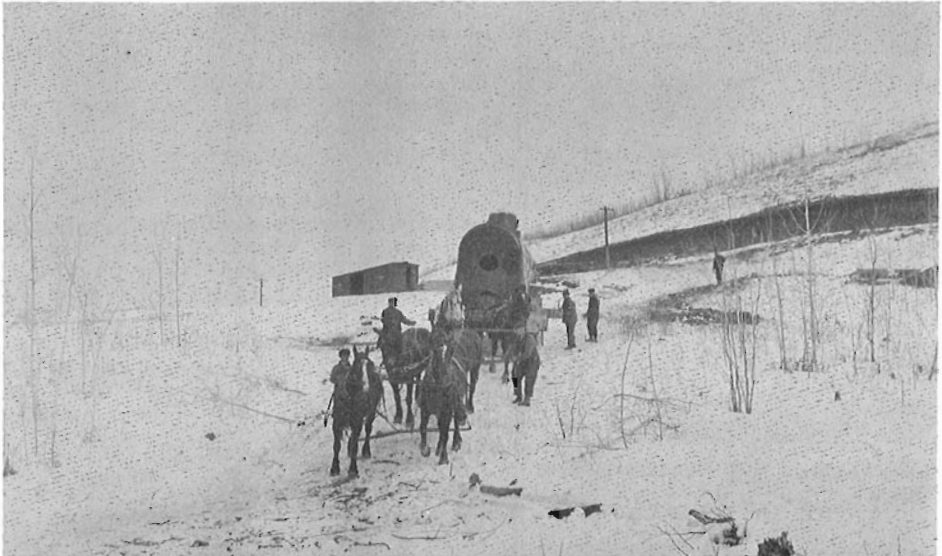
Even the heart of a local Lake Steamer arrived by rail and had to be off loaded onto a team drawn skid . The boiler for the S.S.D.A. Thomas is shown here being eased down the hill from Central Canada Railway at Judah Hill Crossing in 1916. Photo courtesy Mrs. E.Hanson from the collection of Mr. Wm. H.Meikle.
