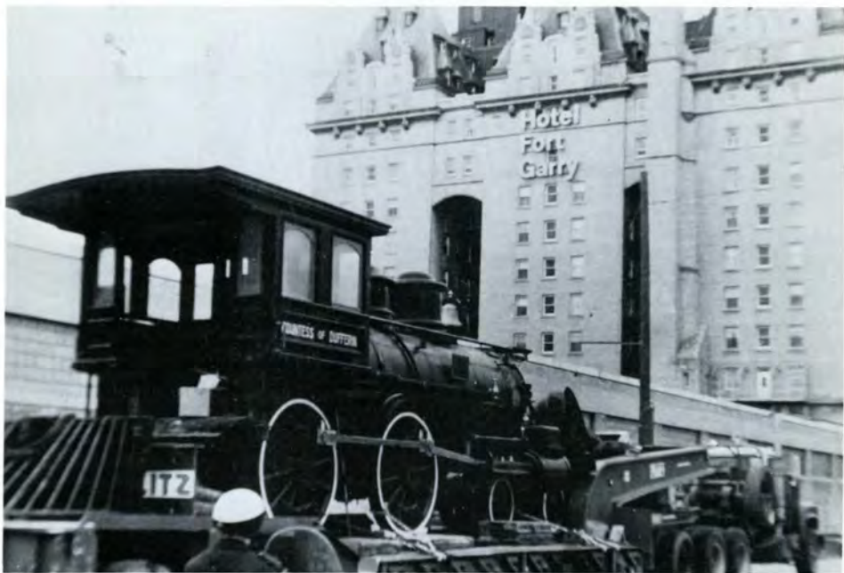
These three photos, all courtesy of the Midwestern Rail Association show the delicate move of the 'COUNTESS' to her new albeit temporary resting place. The locomotive will be permanently displayed in the soon-to-be constructed museum once all the facilities are completed.
