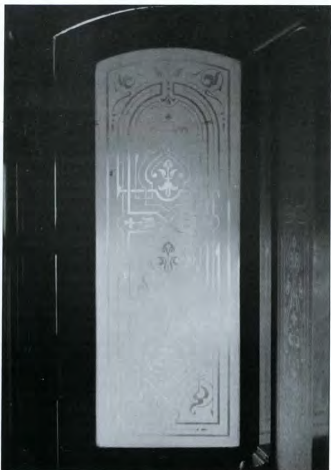
Still intact is this decorative etched glass door leading from the passenger to the dining area of the car.
