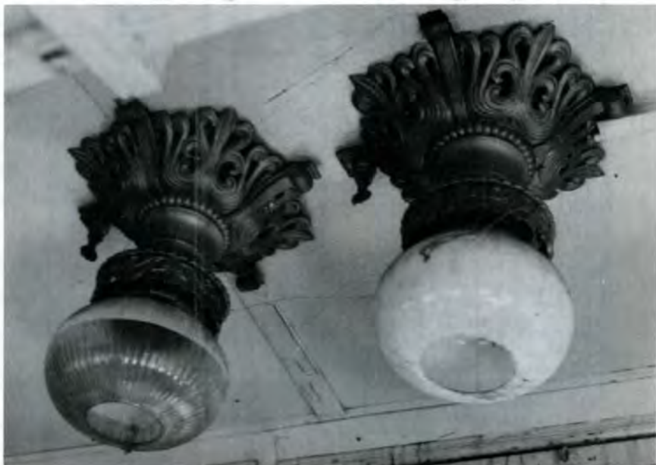
These pintsch gas ceiling fixtures are still in place over the table in the dining end of the car. Note the spider webs admitting to years of peaceful disuse.
