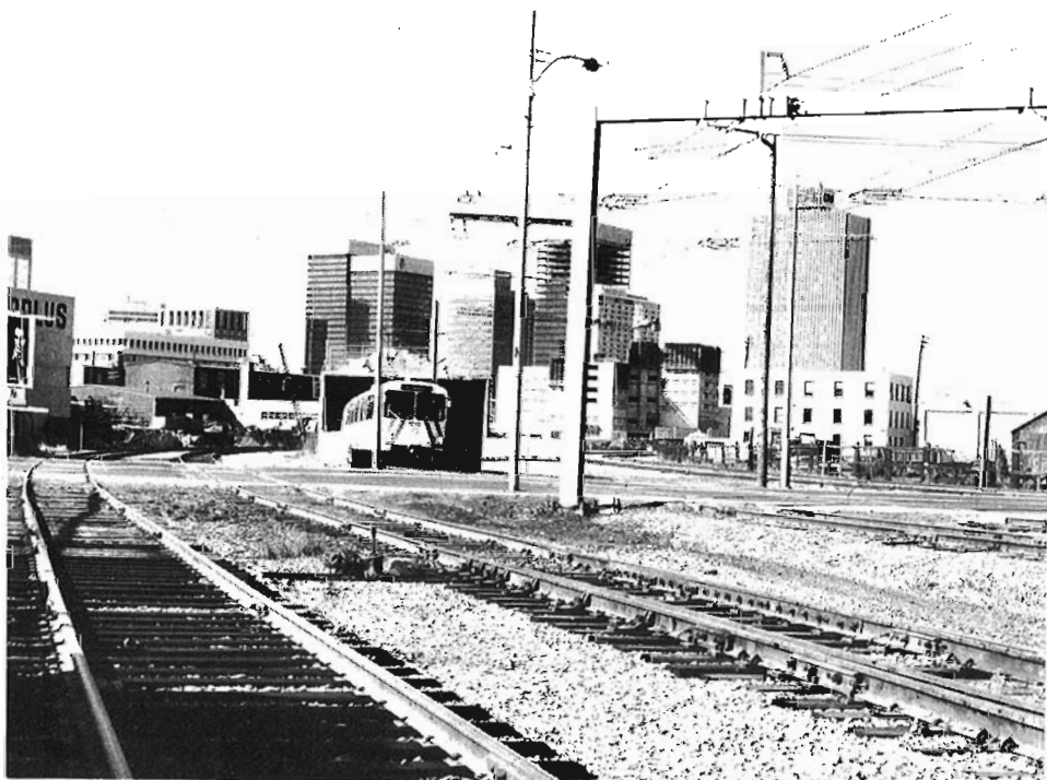
Car 1012 heads a train into the sunlight at 95th. St., CN tracks are on both sides of the LRT at this point. The LRT line terminates 1.6km underground and to the left. Photo courtesy of the authors.
