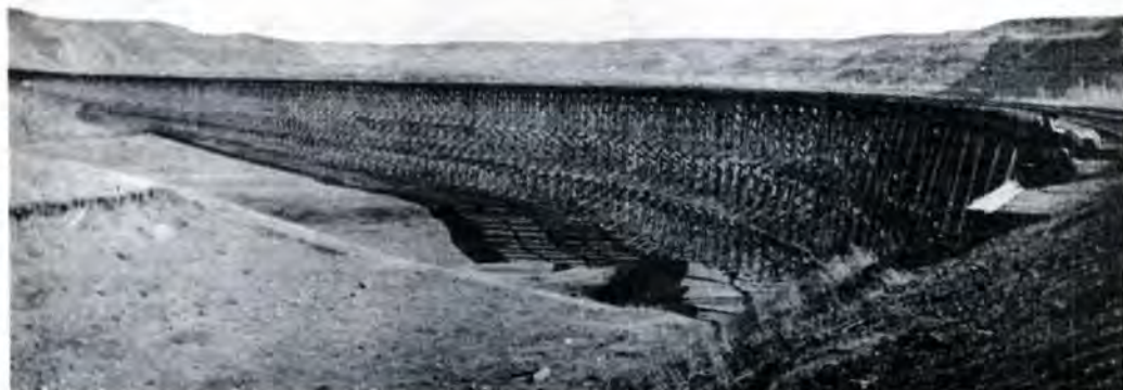
St. Mary River trestle from its west end, the eastern edge of the Blood Reserve.
