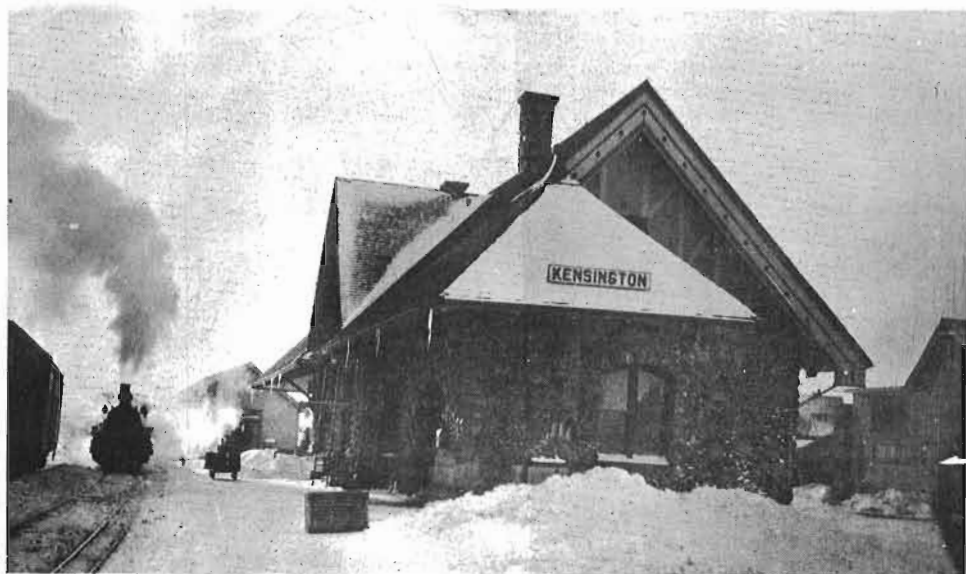
A view of Kensington Station taken while the third rail was being used; a narrow gauge train is coming eastward on the mainline. Photo copied by Margaret Mallett; original in possession of P.E.I. Heritage Foundation.
