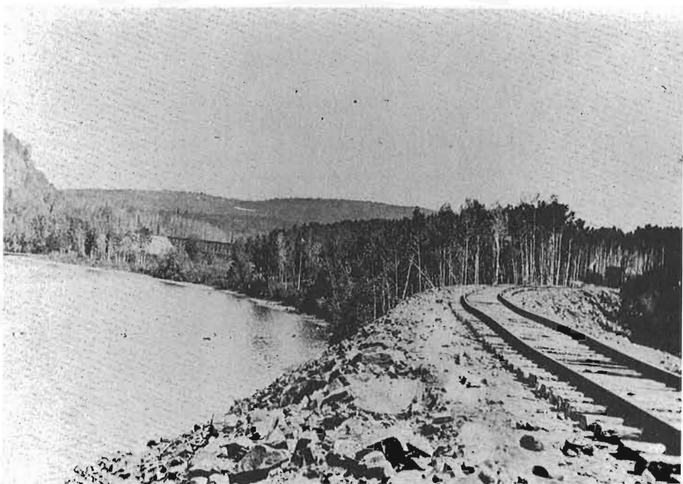
Railway Construction before levelling near Orient Bay, Ontario. Photo courtesy Mr. A.J. Isbester.
