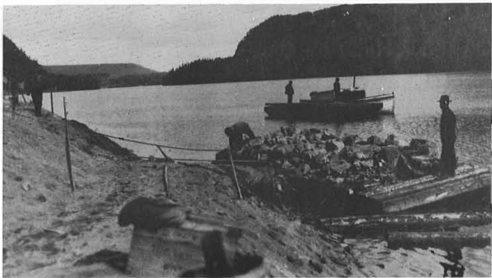
"Riprapping" at Orient Bay, by A.J. Isbester
