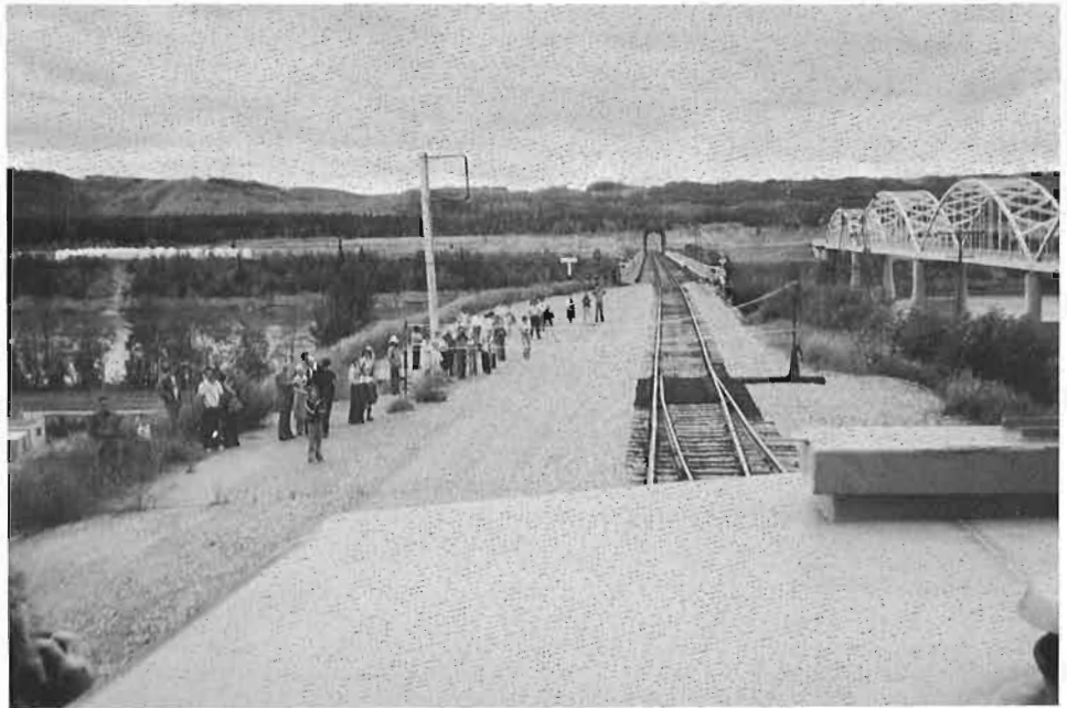
The approach to the bridge, the highway bridge is at the right and was built in 1968, once over we have the view from the other side looking back from DUET.
