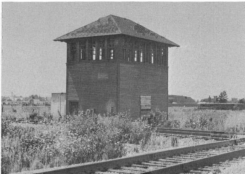
The disused T. H. & B. / CONRAIL tower called E&O Tower, Ont. as it appeared in June 1976. Vandals have not overlooked a single pane of glass.
