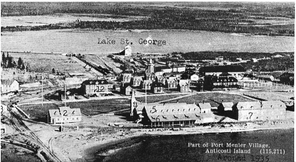
A general view of Port Menier around 1935. Some points of interest are indicated on the photo by numbers: 1 Power House. 2 Company's office. 3 Car Shed. 4 Roman Catholic church. 5 General Store. 6 Meat market and cold storage. Track passed underneath snow shed. 7 Main warehouse. 8 Hotel. 9 Club room. 10 Village water tower. 11 Engine house and engine repair shop. 12 Convent. 13 Port Menier canal (man made).
