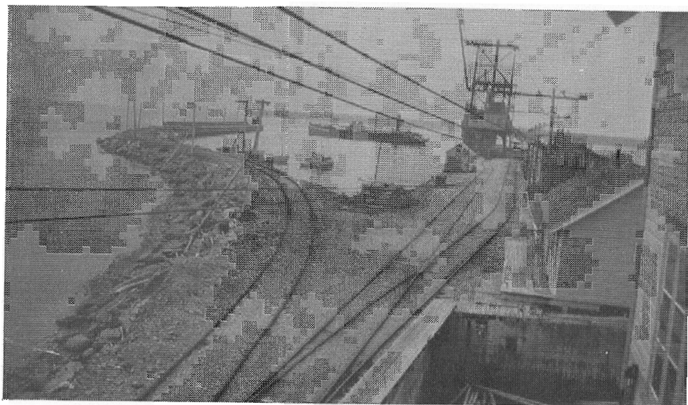
The tracks at the end of the wharf and on the breakwater about 1922. Collection, Roger Samson.
