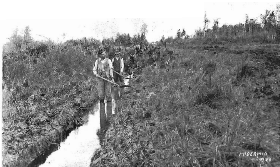
MEN DIGGING THE DRAINAGE DITCH beside the cleared right-of-way. October 1913.
