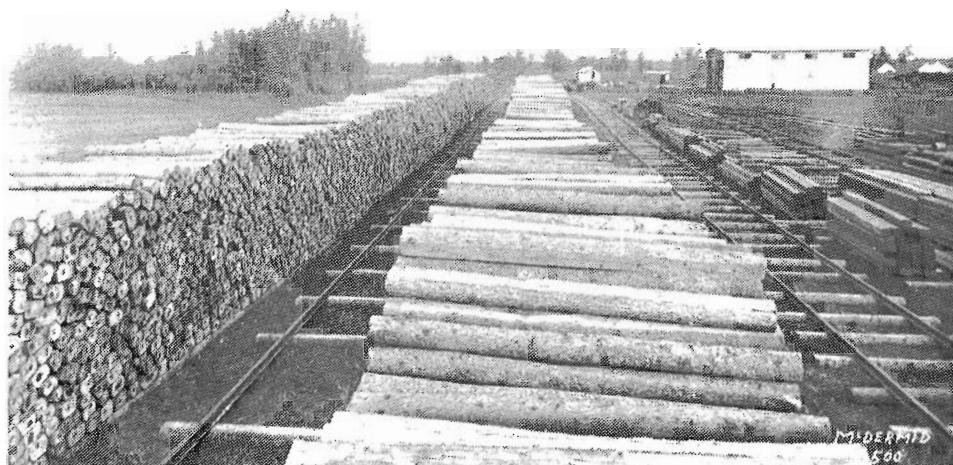
PILES OF NEW TIES IN THE YARD of the Edmonton Interurban during the construction of the line in October, 1913.
