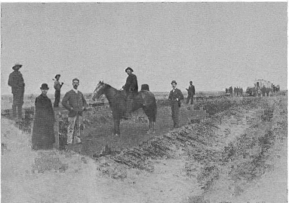
The A.R. & C. Co. track near Lethbridge, Oct. 1, 1890. There is some grading under the track, however, just behind the right hand figure, it is on the virgin prairie. The furrow in the foreground acted as a sometimes ditch, and at first, until overgrown, a firebreak from the periodic grass fires which ravaged the area. (Author's Collection)
