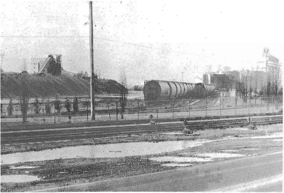
NORMAL CONDITIONS AT NEPTUNE show stock pile of export coal and tank hopper cars on the unloading circuit track
