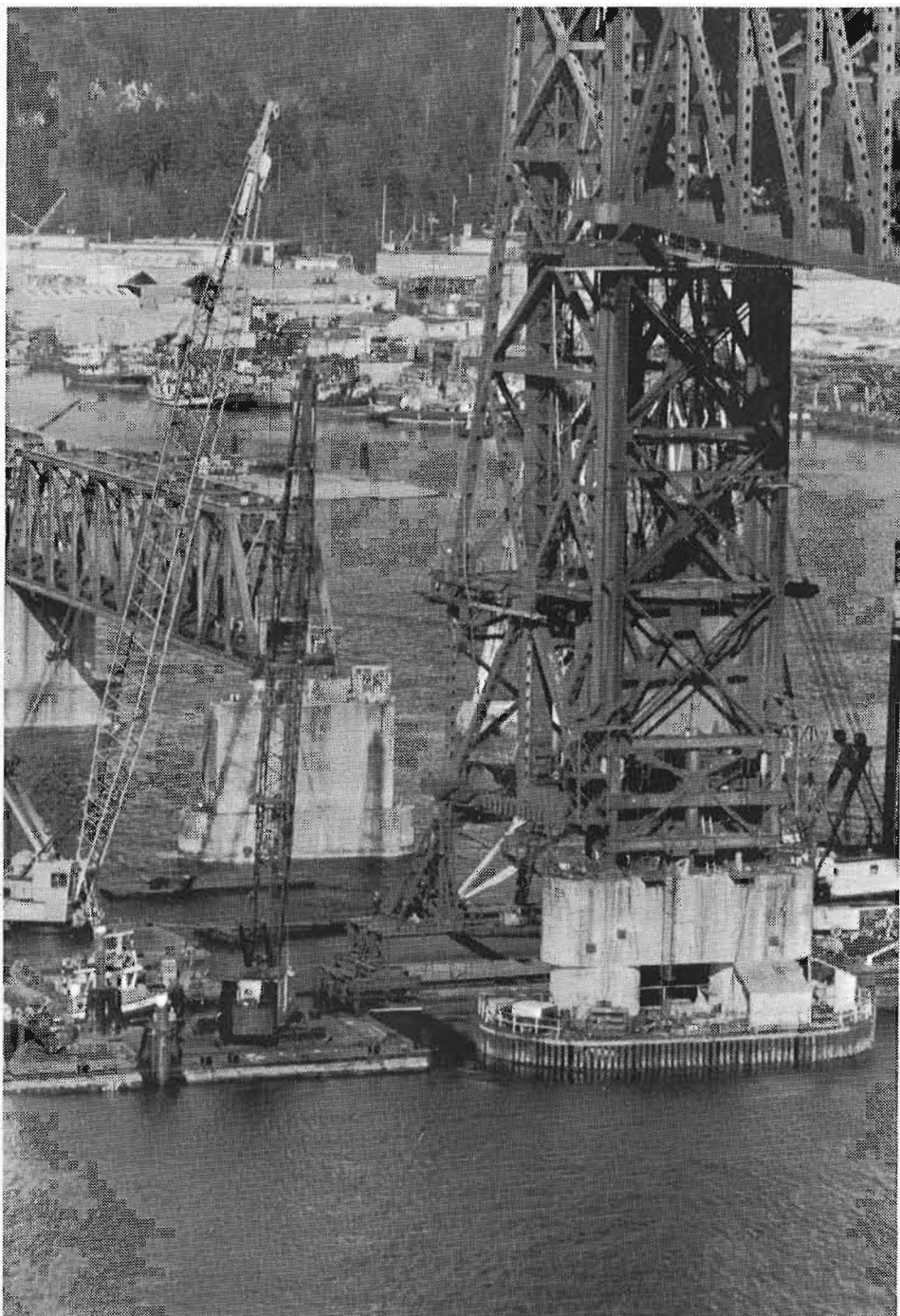
DAMAGED SPAN REMOVED for repair and strengthening.
