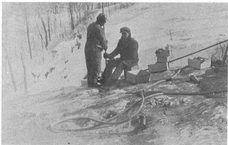
LOADING DYNAMITE INTO THE DRILLED HOLES in preparation for blasting for the cut at the East end of the tunnel. The sun is shining but the weather is cold as work continues in March 1928.
