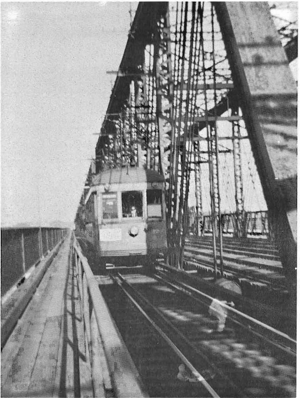
A RATHER RARE VIEW showing the M. & S.C. track on Victoria Bridge with car 320 approaching Montreal in 1949. What is now the downstream roadway on the bridge was then shared by the electric line and a sidewalk for pedestrians and bicycles. The main C.N.R. tracks are in the background inside the span.
