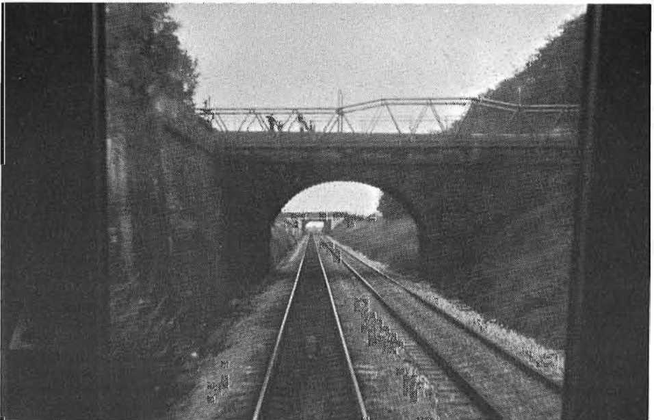
GOING UP THE SUTTON INCLINED PLANE the train is about to pass under the New Street bridge, one of the original L. & M. bridges built in 1829. This is one of the 1% grades which it was feared could not be surmounted by locomotives, until the "Rocket" proved this fear to be groundless. The bridge is still in use, but as it is only 26 feet wide it has had a rather ugly modern sidewalk attached to one side.
