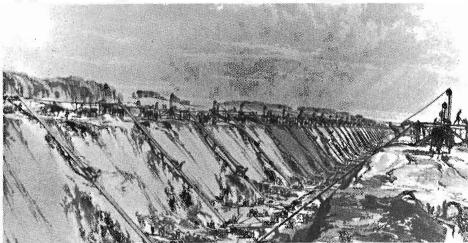
ONE OF THE MOST FAMOUS VIEWS BY J.C. BOURNE shows the excavation of Tring cutting just north of London in 1837 during the building of the London and Birmingham Railway. The entire cutting was dug by hand, the earth being hauled out by means of wheelbarrows.
