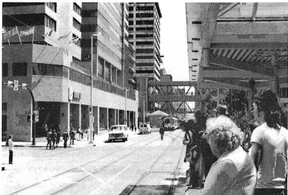
THE FIRST REVENUE TRAIN ON THE CALGARY SYSTEM waiting at the next-to-last station in downtown Calgary. The first passengers are waiting in the foreground. Rick Shantler.
