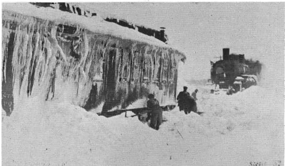
THESE TWO PHOTOS DATE FROM 1909 and show the effects of snow on passenger trains. One view is captioned "The first train through Jan 31 09" and the other depicts efforts being made to free an open-platform wooden postal car from a drift.
