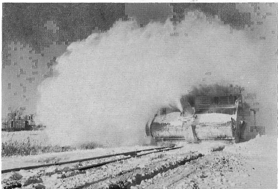
SNOW CLEARING IN YARDS is now done by modern snow blowers like this unit shown at work in St. Luc yard in January 1966.
