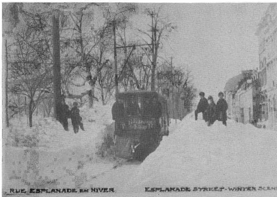
RUE ESPLANADE, Quebec City in the 1890's. Sweeper 4 has just passed through a large drift as local youngsters look on. Public Archives of Canada PA 31907.
