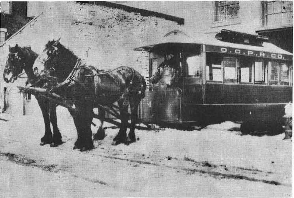
ANOTHER RELIC OF THE HORSE CAR ERA to survive is Ottawa City Passenger Railway car 4. Ottawa also used sleighs in winter, but this shows a regular horse car as it would appear during early-winter or early-spring operation. However this photo was taken much later as can be seen by the absence of a truck under the car,
