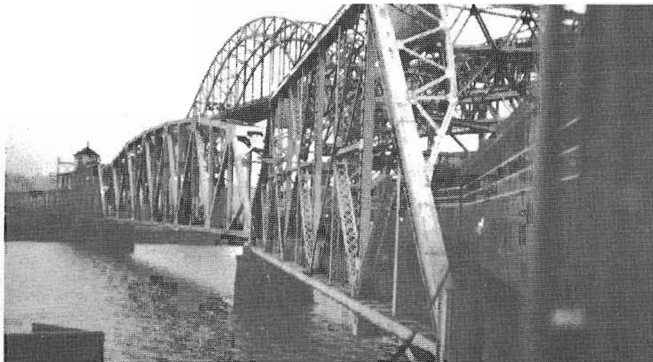
Approach to the New Westminster Fraser River rail bridge.
