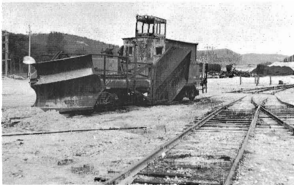
SNOWPLOW OF THE KILMAR - MARELAN RAILWAY. Simple but effective.
