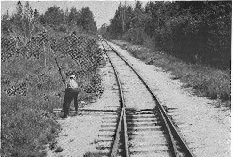
THE END OF THE "TWO MILE STRAIGHT" showing the switch into the Y adjacent to the main line connection.
