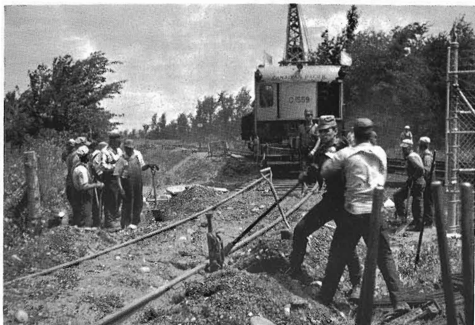
TWO VIEWS OF THE C.P.R. TRACK GANG building the siding into the museum property on July 10 1962. Note that the building is now sheathed.
