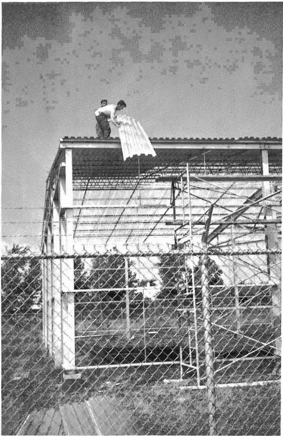
THE FIRST ALUMINUM SHEATHING goes up on building 1 on June 21 1962.
