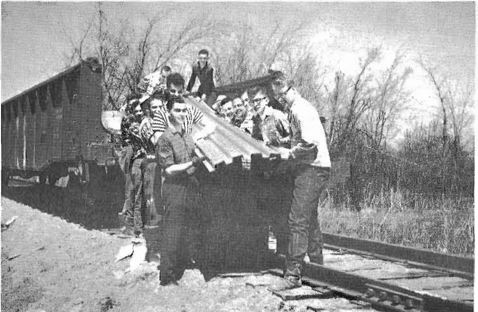
A GROUP OF VOLUNTEERS unloading a flat car on the Candiatic spur on May 12 1962. The load is the aluminum sheathing which was soon to be placed on building No. 1.
