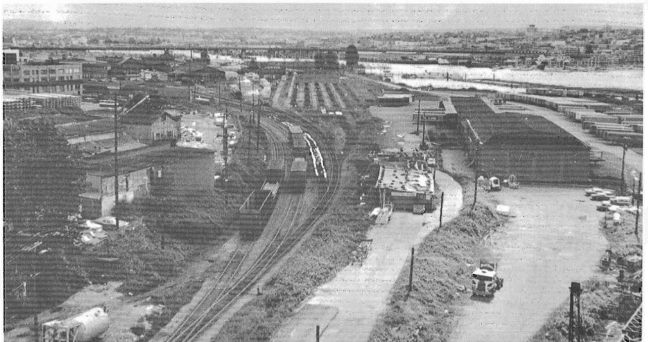
Drake St. yard looking east towards the Cambie Bridge, after 9 storage tracks have been lifted. Shown is the point where C.P. & B.C.E.R. would exchange cars. Photo courtesy of Norris Adams, Vancouver
