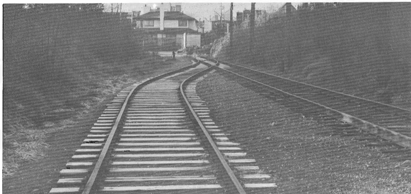
Old Kitsilano carline now shortened to end at the barrier at Chestnut Street. A house now stands astride the former right-of-way, ahead. This is just one city block from the Kitsilano car shops-now being demolished.
