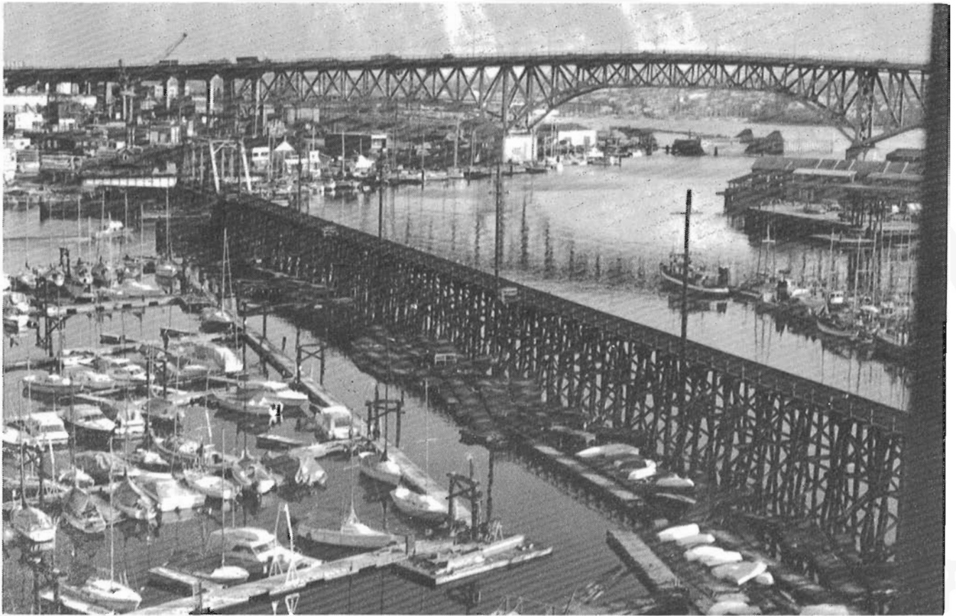
Pictured from the adjoining Burrard bridge, looking northeast toward the fixed span. The moveable span is seen open for navigation — a characteristic position. The demolition was done carefully, and stringers, ties and piles were saved. The third Granville Bridge across False Creek looms high in the background. Trolley & diesel & gas busses have used it for 35 years, but no provision was foreseen to use street cars.
