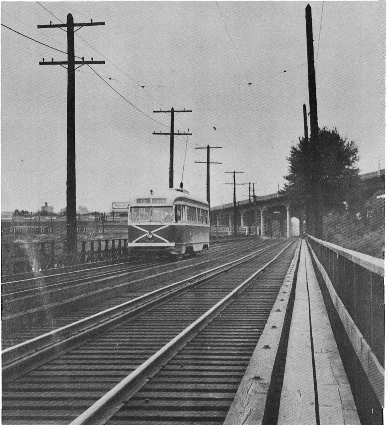
Kitsilano trestle looking south with Burrard St. Bridge in the background. Vancouver 1947. Note the array of trams and street cars in the background and outside the Kitsilano Shops, and also that the line is double-tracked. The piles under the track bed where P.C.C. 408 is shown are believed to have been of Australian long-lasting wood -- possibly gumwood. The car is about 7½ city blocks from the loop at Yew Street, double tracked and high iron. Photo courtesy of Norm. Gidney, Burnaby, B.C.
