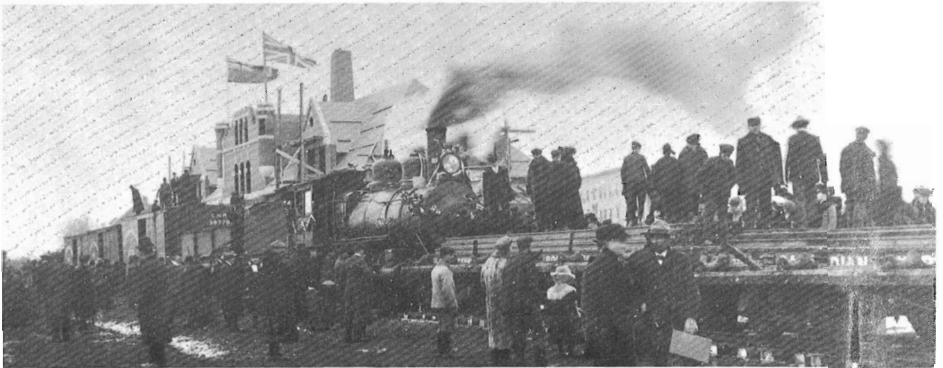
The Grand Trunk station in Edmonton was still under construction when the first train arrived on November 4, 1905. Provincial Archives of Alberta, E. Brown Collection No. B7071.
