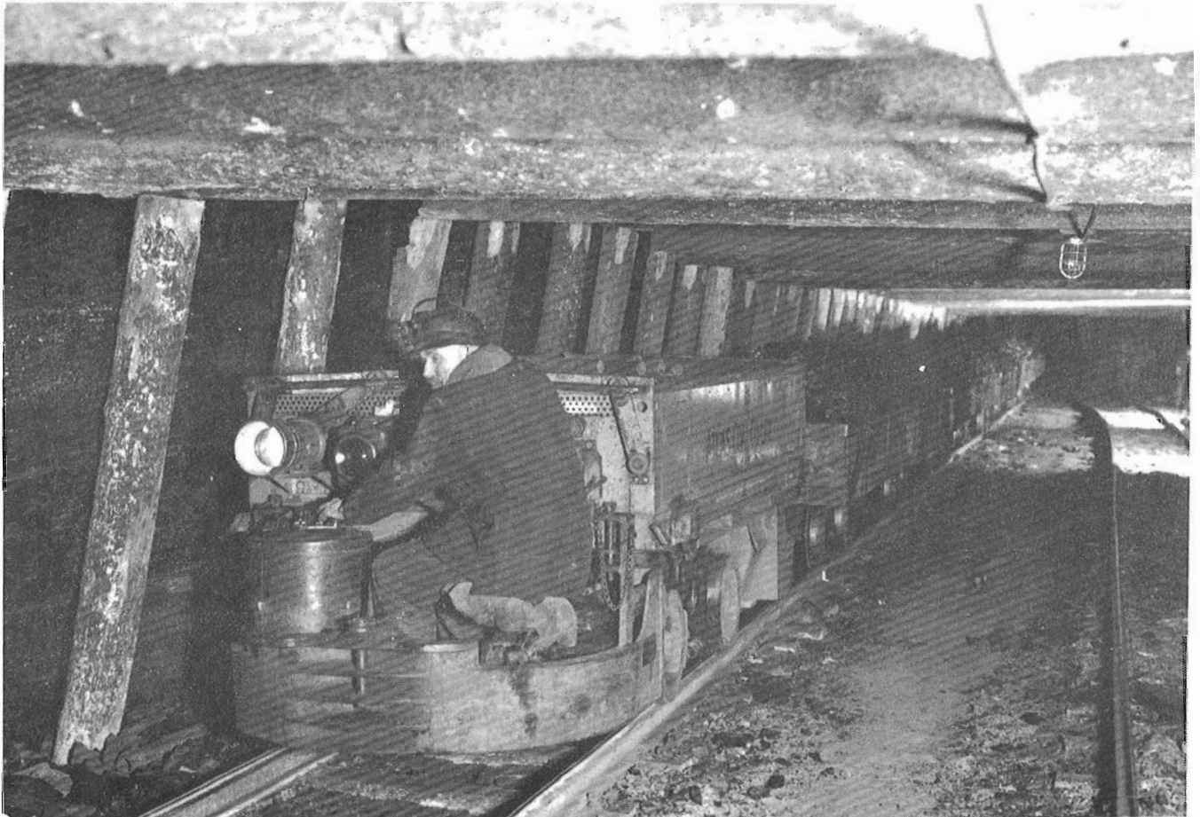
There were many underground battery locomotives such as this one in use throughout the mines in the Drumheller Valley. This one is being used in the Commander Coal Mine at Nacmine on Nov. 29/44. Nacmine is approx. 5 miles west of Drumheller.
