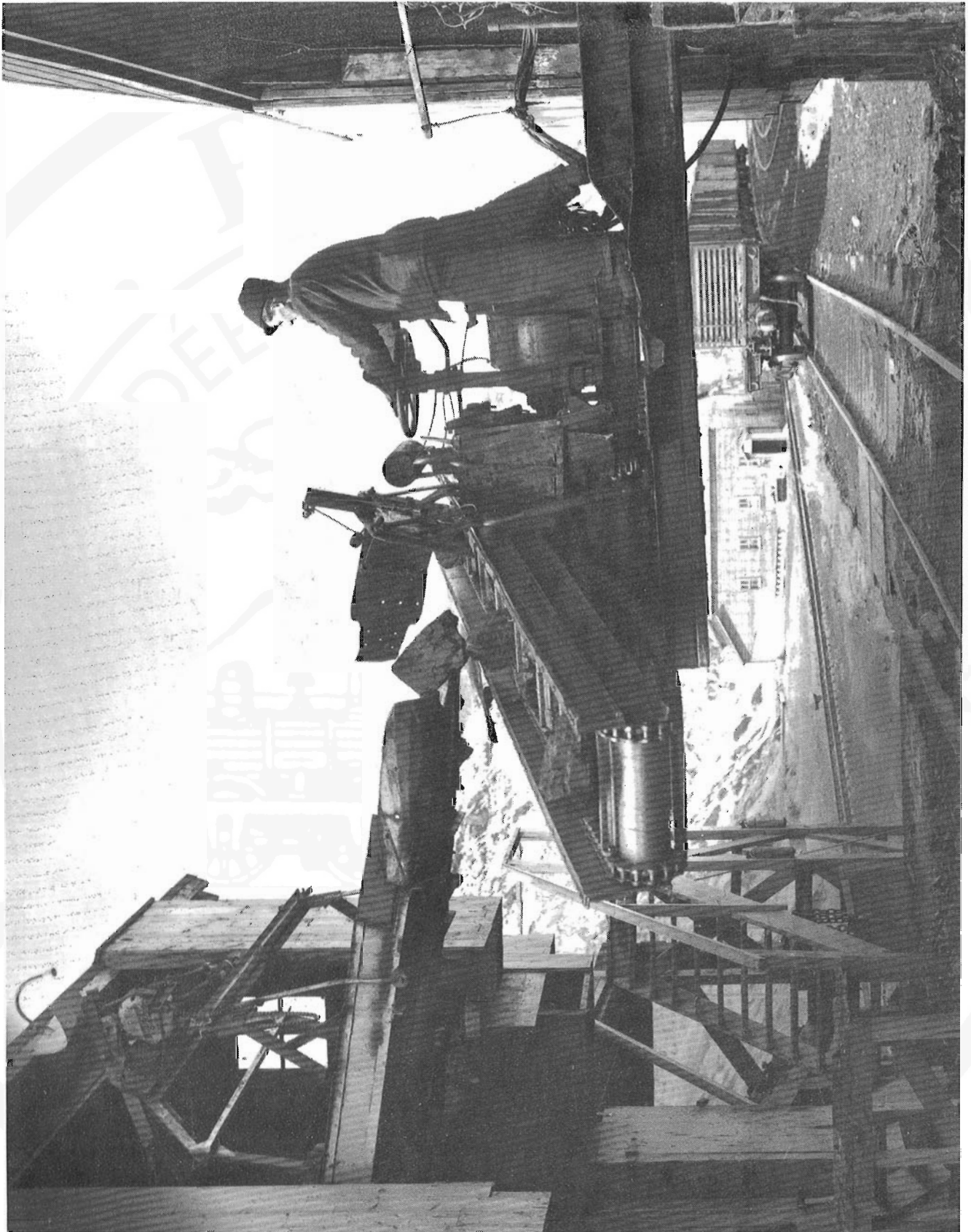
In this 1948 view, an employee of the Atlas Coal Mine prepares to load the waiting cars in the background with this mechanical boxcar loader. P915 Atlas Coal Mine East Coulee, Alta 1948.
