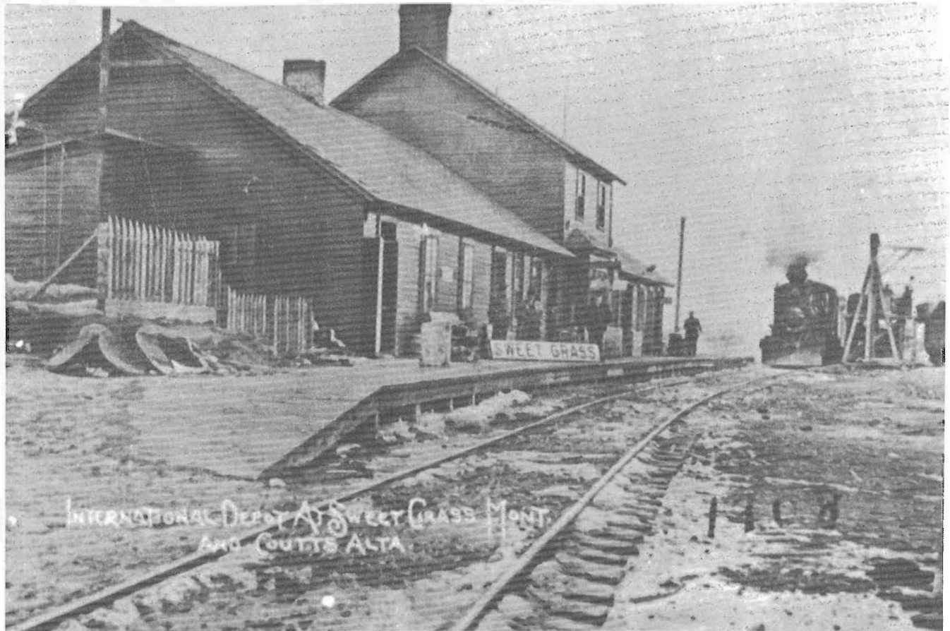
The international station at Coutts seen from the U.S. side, with the Sweet Grass station board propped up on the platform. A narrow gauge engine takes on coal from a bucket loader, the water tank is in the immediate right foreground as evidenced by the ladder.
