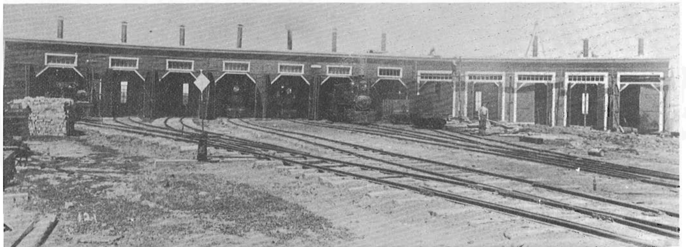
The Lethbridge roundhouse not yet finished, probably in 1890 about the time trains began running over the new tracks. The last three stalls at the right are still incomplete.
