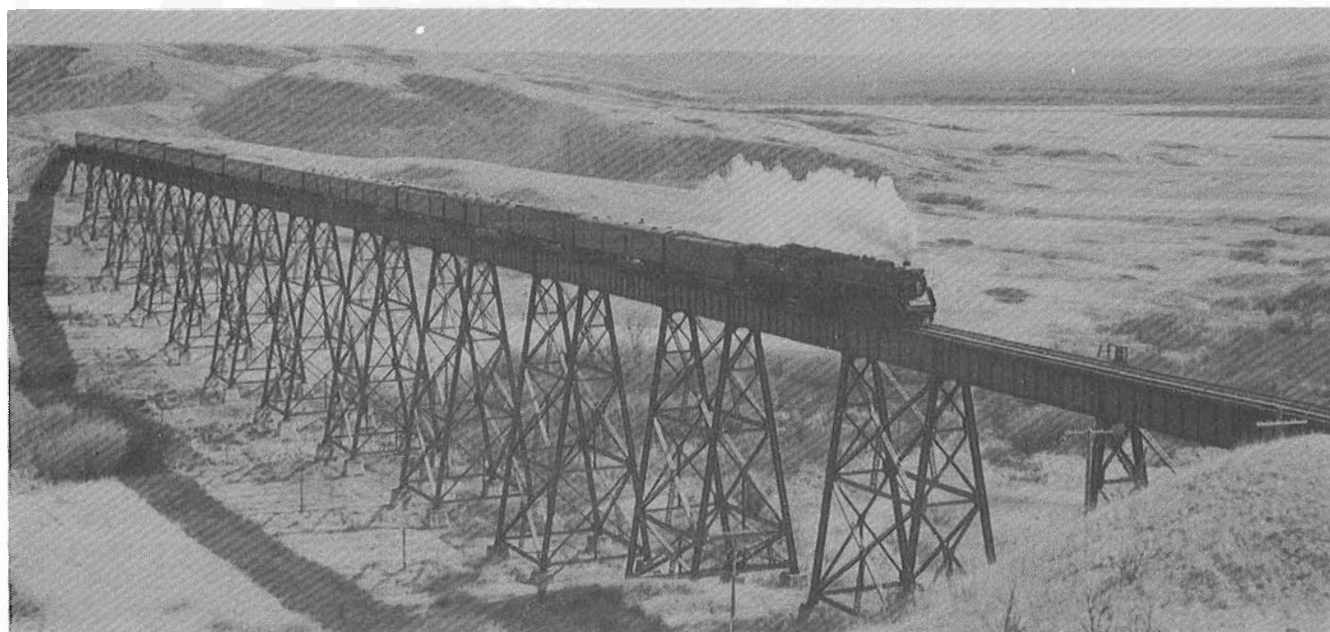
The longest bridge on the division is the present Uno trestle, opened by the CNR in 1929. It is 1,583 ft. long with a maximum height of 116 ft.. On May 6, 1954 class U-2g 4-8-4 6210 is wheeling 15 coaches of No. 3, first section of the Continental Limited. In 1954 the 6207, 6210 & 6211, replaced by deisels on eastern lines, made occassional trips in place of 6000's on this division. The next year all passenger service had diesel power. There have been no passenger trains since withdrawl of the Super-Continental on Nov. 15, 1981. L.A. Stuckey photo
