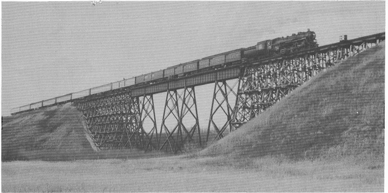
By 1924 the original Rivers trestle had been filled in all but 640 feet. That year CNR built a new steel center section, 250 feet long with 91 feet maximum height. With strengthening of timber approaches the bridge would remain in this form until 1970. Engine 6057, a class U-1e 4-8-2 is getting under way with 11 coaches on No. 4, second section of the Continental Limited on Nov. 1, 1953. L.A. Stuckey photo
