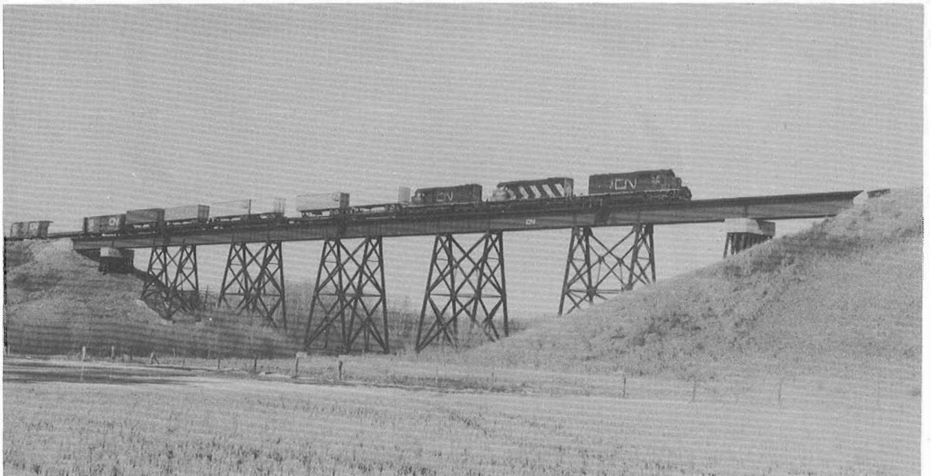
By 1924 the original Rivers trestle had been filled in all but 640 feet. That year CNR built a new steel center section, 250 feet long with 91 feet maximum height. With strengthening of timber approaches the bridge would remain in this form until 1970. Engine 6057, a class U-1e 4-8-2 is getting under way with 11 coaches on No. 4, second section of the Continental Limited on Nov. 1, 1953. L.A. Stuckey photo
