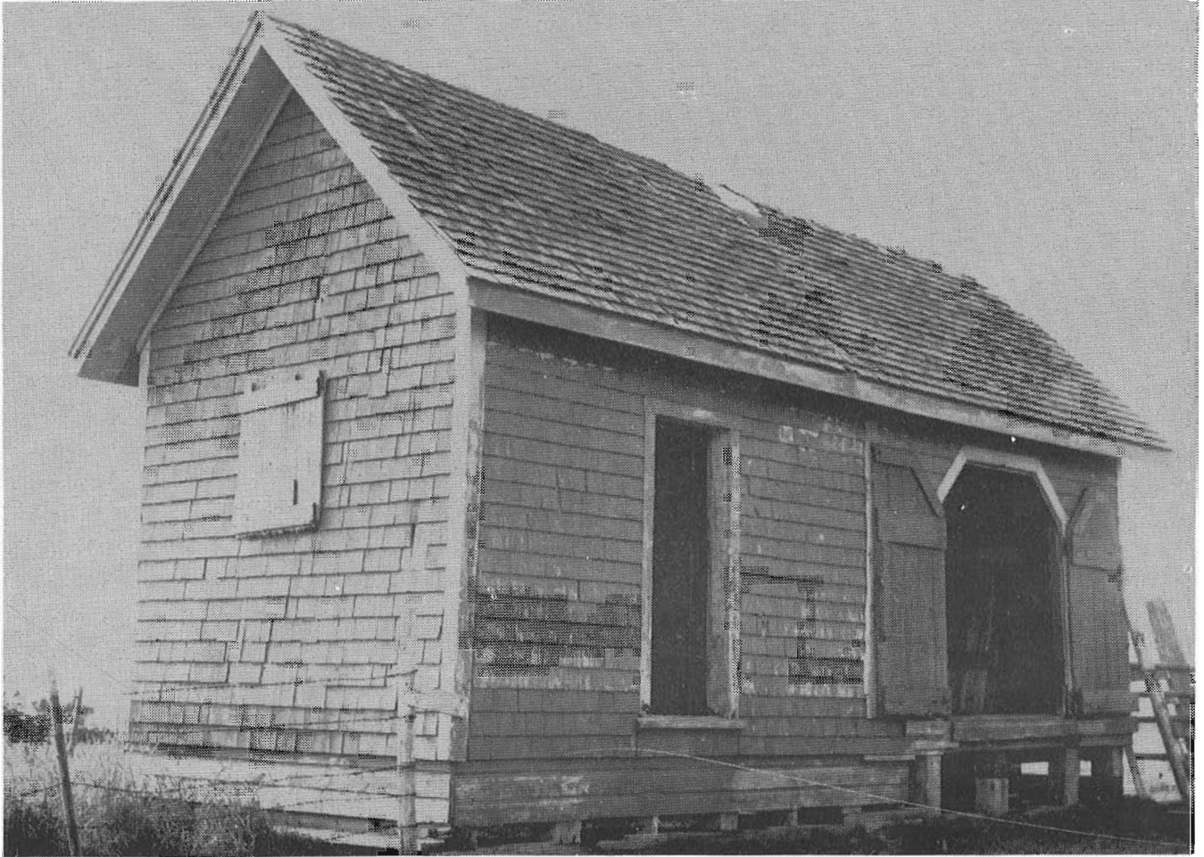
Colville station, now used as a farm storage building. (Margaret E. Mallett photo).
