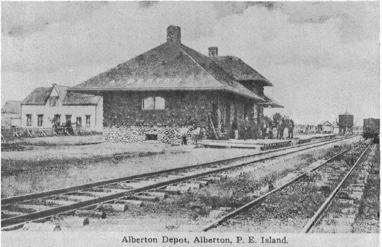
Postcard showing the second Alberton station built of boulders in 1905. Note the water tower at the wye. (Copied by Margaret E. Mallett from an original in the collection of the P.E.I. Museum and Heritage Foundation).
