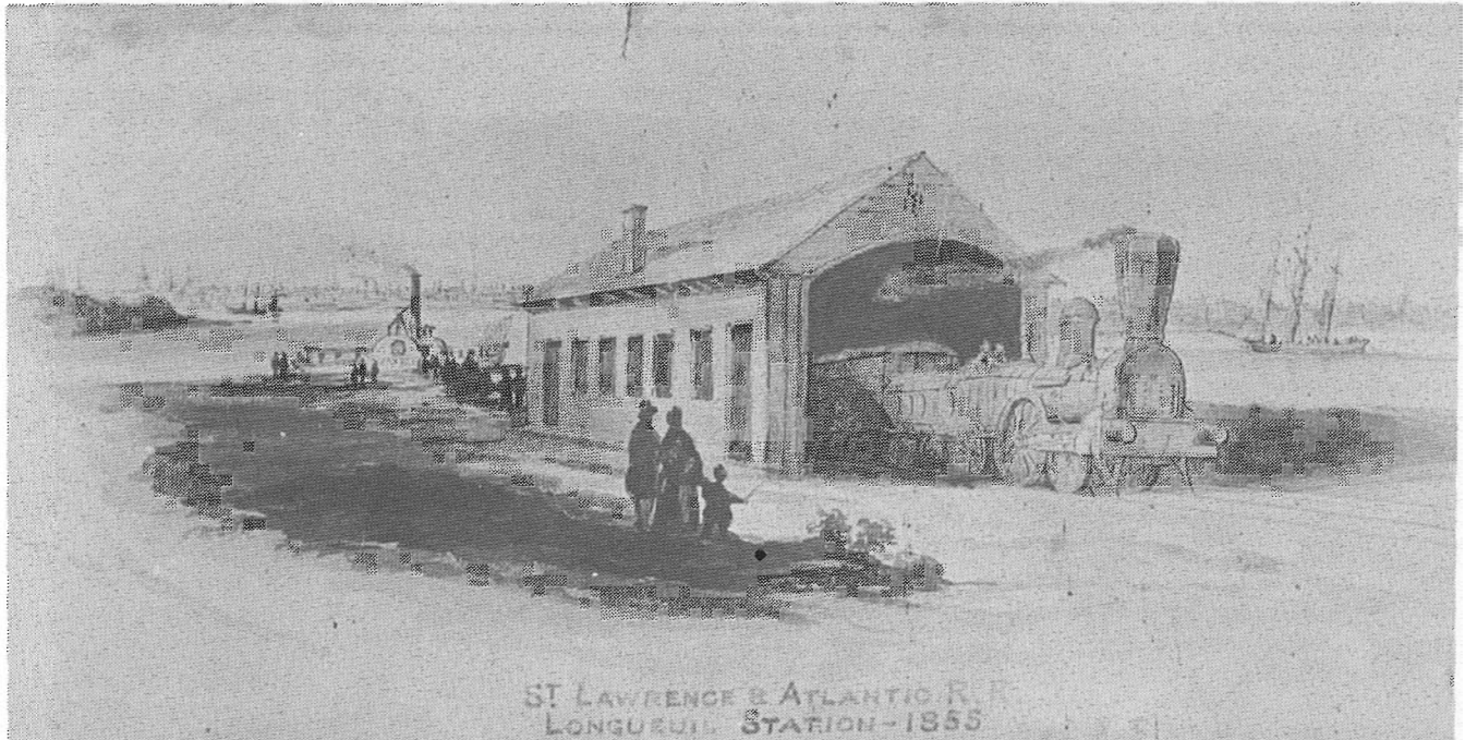
FIGURE 3. THE WASH DRAWING OF LONGUEUIL WHARF STATION of the St. Lawrence and Atlantic Railroad in 1855. The 2-2-2 locomotive is the "BRITANNIA" which came second-hand from Scotland in 1848. This appears to have inspired the locomotive in the Walker drawing.
