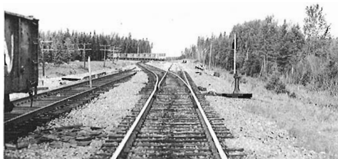
Pelletier Station; - The switch is in normal position for Monk Sub. This photo at the same location that no 63-14A.
