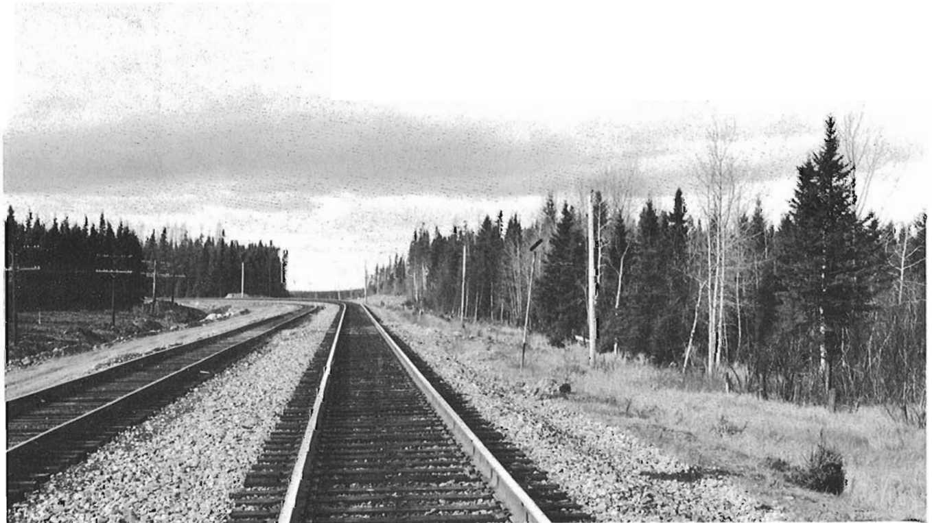
Pelletier Station; - Looking west. In the curb, we see the clearing after the woodcutting, in a few years, the curve will be no more
