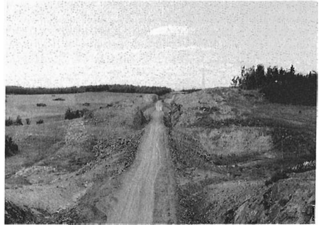
On concession road 5, viaduct looking west, we see the Riviere-du-Loup Bridge.
