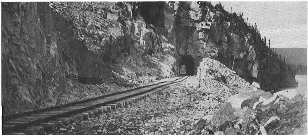
Final Obstacle: Jack Fish tunnel in the spring of 1885 showing the newly laid but unballasted main line over which the garrison artillery's troop train moved to the driving of the last spike in the east. Buell Photograph; Omer Lavallée collection.
