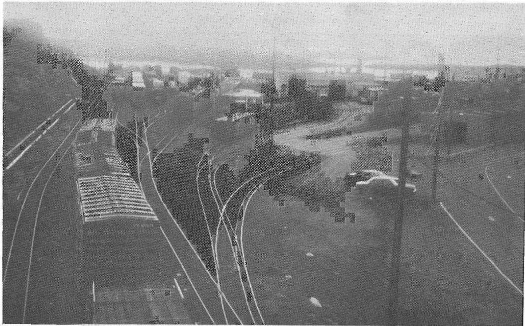
The Terra Transport yards at Port Aux Basques. Note the dual-gauge track.
