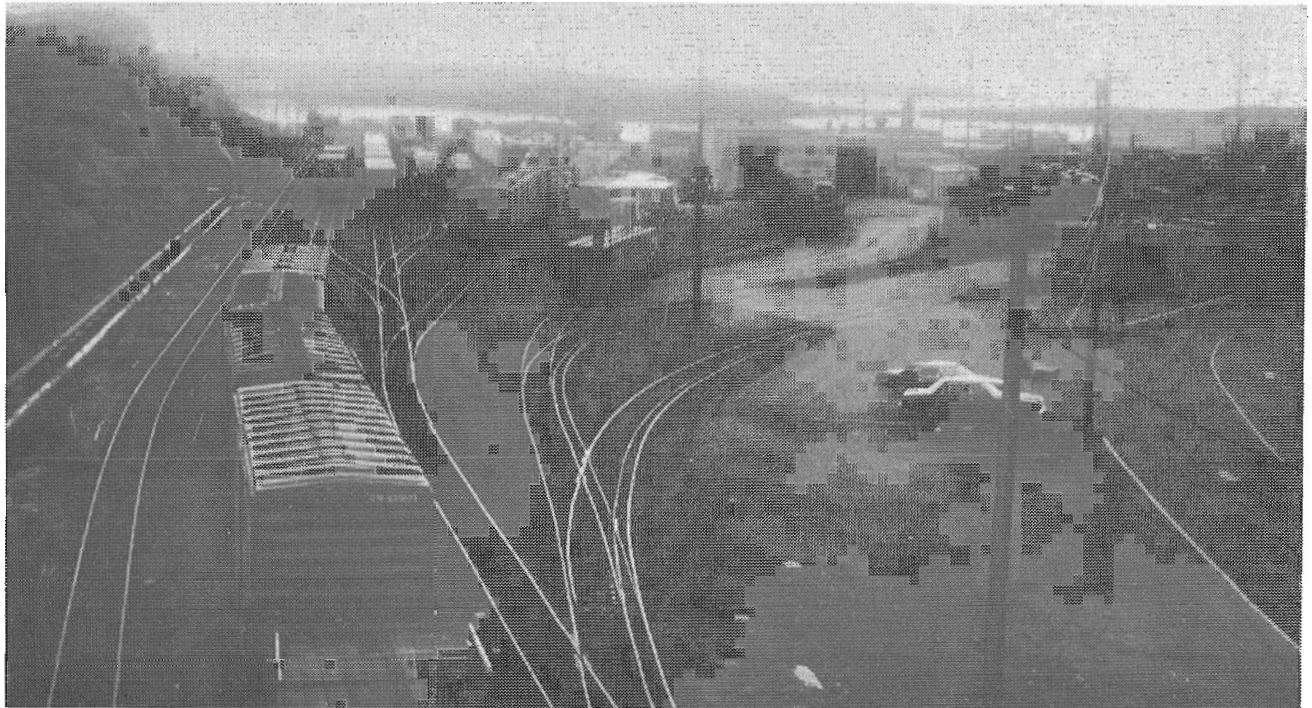
A dual-gauge yard at Port aux Basques in Newfoundland. Here the two gauges come together and car bodies are transferred from standard-gauge trucks to narrow, and vice versa. Photo by Fred Angus.
