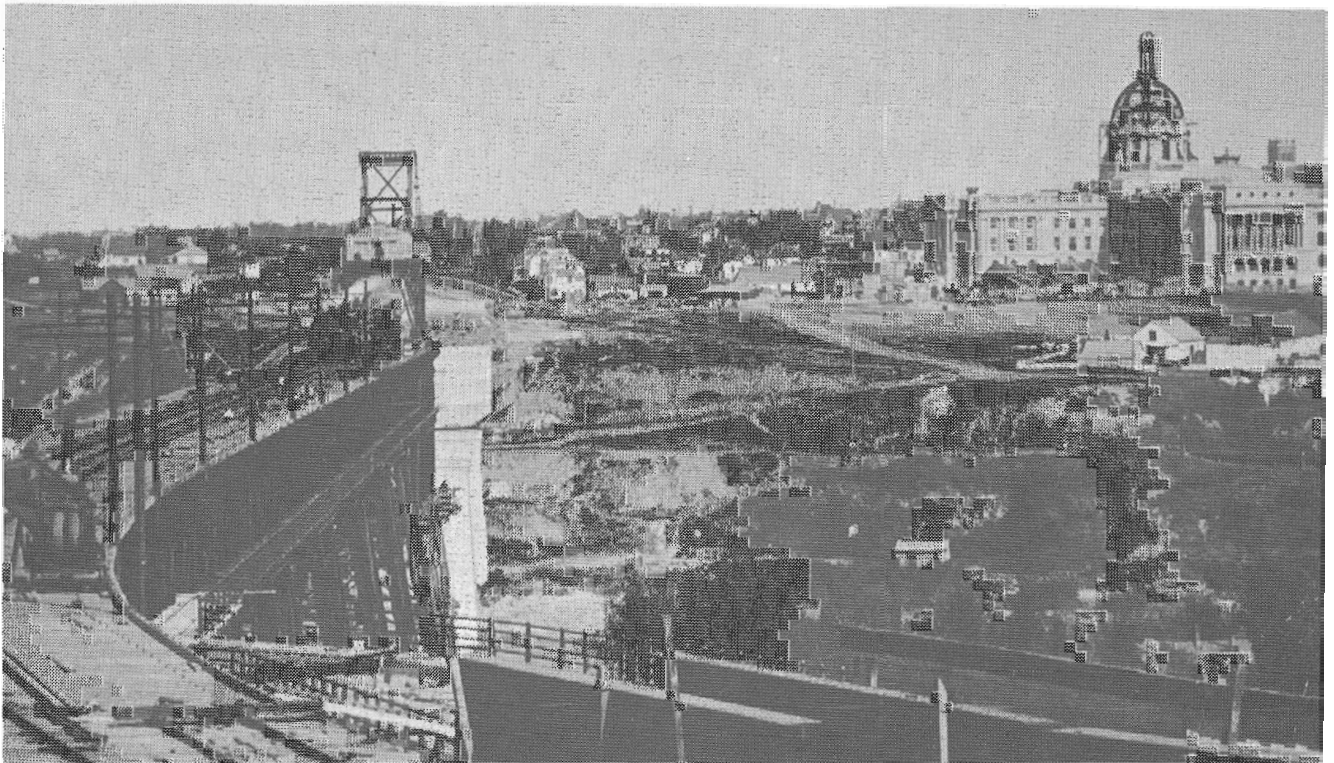
Canadian Pacific High Level Bridge under construction. It also shows some of Fort Edmonton buildings on the grounds of the Parliament Building with the dome still being constructed.
