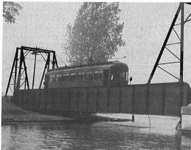
Chambly swing bridge CN photo.
