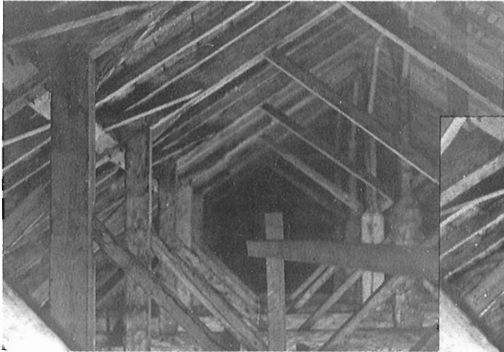
Inside the attic of the building, showing the roof bracing typical of the construction used in the first half of the 19th century.
