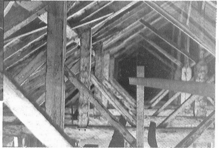
Inside the attic of the building, showing the roof bracing typical of the construction used in the first half of the 19th century.
