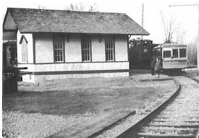
Barrington station on its new foundation. David Johnson.
