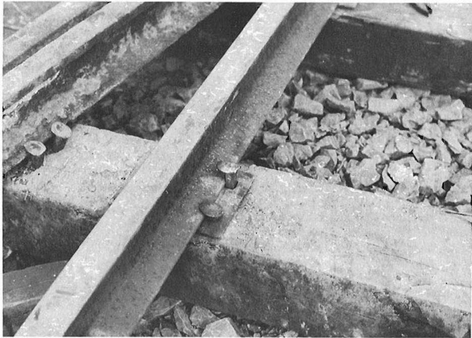
The "last spike" on the new tramway line. David Johnson.
